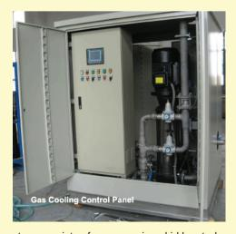
The system consists of one pumping skid located ground level and one regulating skid located at lance elevation. Pump skid is instrumented with multi-stage pump, pressure gauge, Programmable Logic Controller (PLC) for auto on/off. The regulating skid consist of air and water automatic regulating valves, compressed air dryer, manual valves, purge line etc. Lance nozzle tipe is constructed of Hastelloy C22 material to withstand the corrosive operating conditions.
